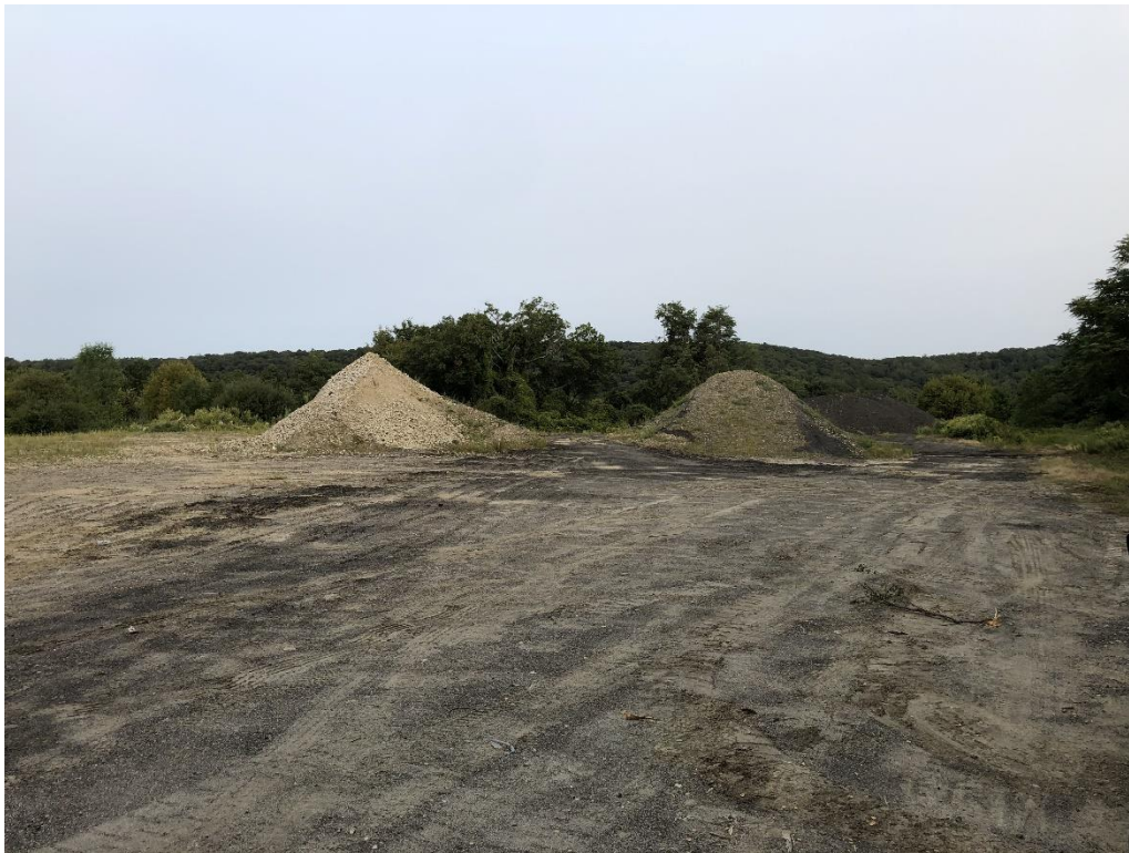
Photo 4. General view of staging area facing north.
